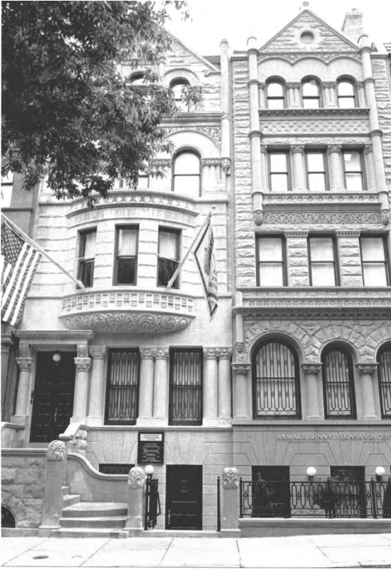
The restored façade of the Center's buildings
